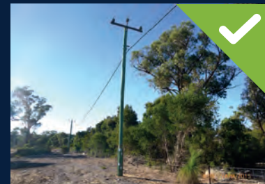
Compliant: cleared buffer zone around power poles
