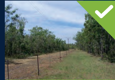
Compliant: grass slashed to ground level
